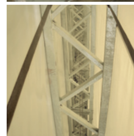
1. Argano a funi / Winch with cables 2. Cinghie di sollevamento e vista delle traverse intermedie a struttura metallica tralicciata / Lifting belts and view of the metal truss structures of the middle cross-pieces
